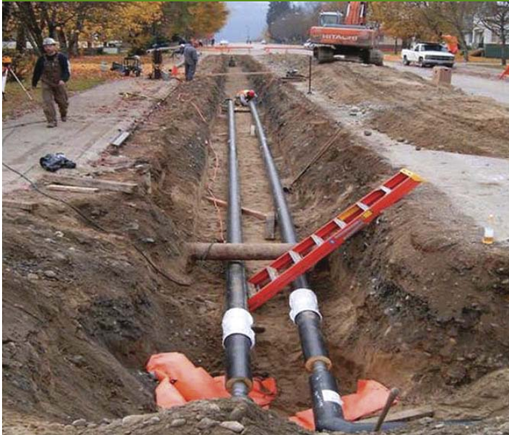
Steel pipes were installed as part of Revelstoke's district heat system. (Photo: Revelstoke Community Energy Corp.).
